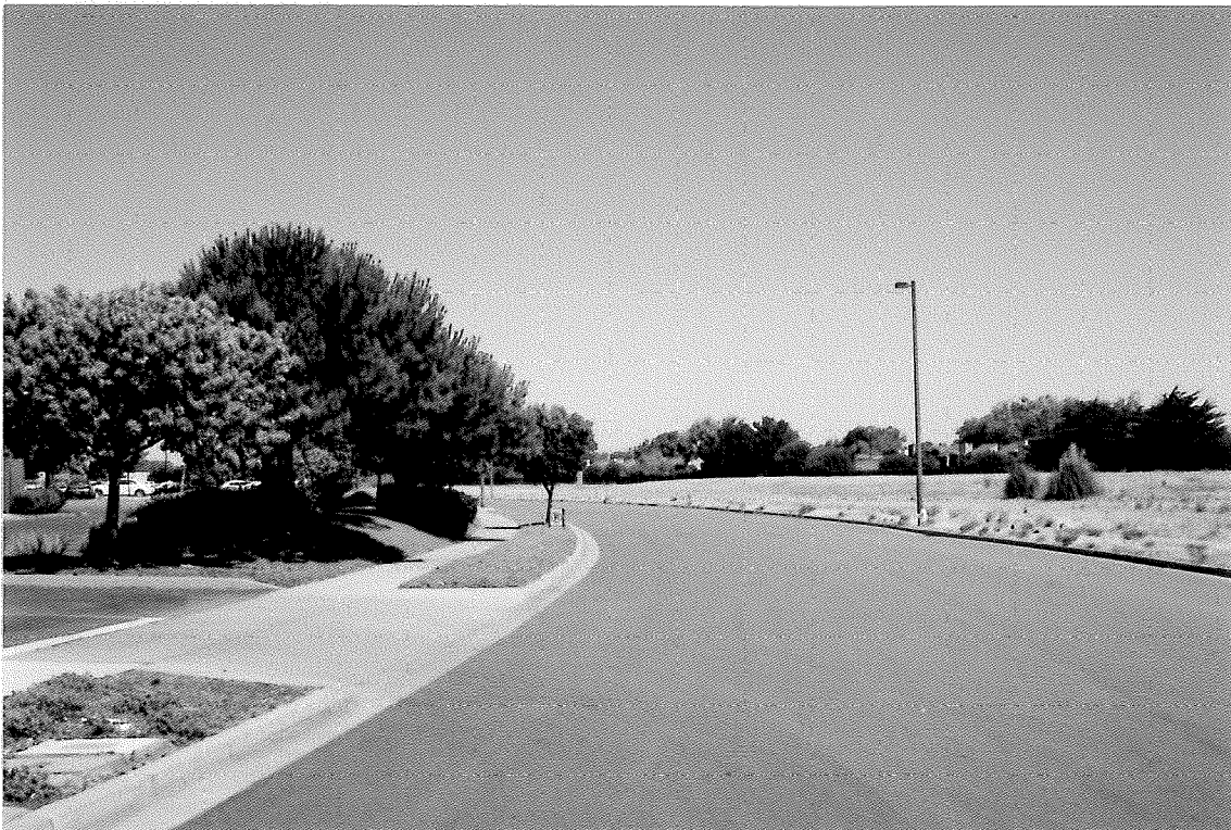
(2) North Loop Road, looking west
